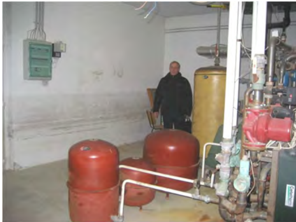
Picture of damage to equipment
